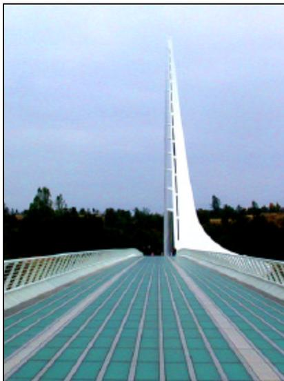
*The pedestrian walkway is of glass and granite. The cables protrude through the deck to anchor to the steel below.*
