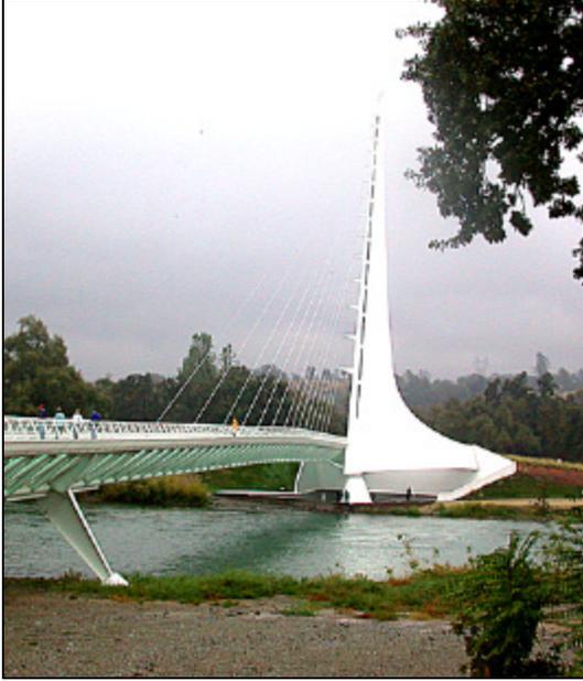
*From a vantage point east of the span, it is evident that the construction pays homage to its natural setting. Ducks, salmon, and small fishing boats have free rein. The pylon is 217 feet tall, measured from its ball-bearing support at river's edge.*
