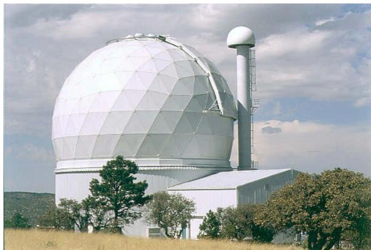
*The mushroom outcrop on the dome houses the laser-alignment equipment that controls the precise shape of the 91 mirror segments which comprise the primary of the Hobby-Eberly telescope at the McDonald Observatory.*
